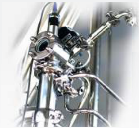
Automatic mechanical seal lubrication with steam condensate loop
